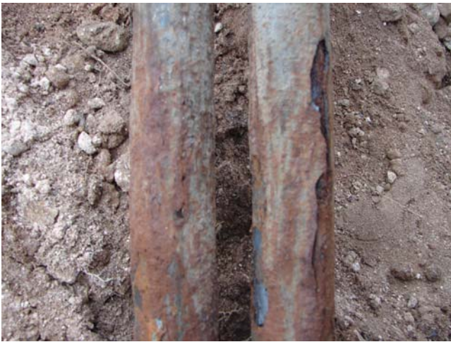
Close-up (2 Foot Below Ground Level)
