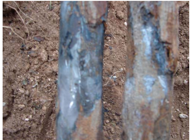
Close-up (2.5 Feet Below Ground Level)
