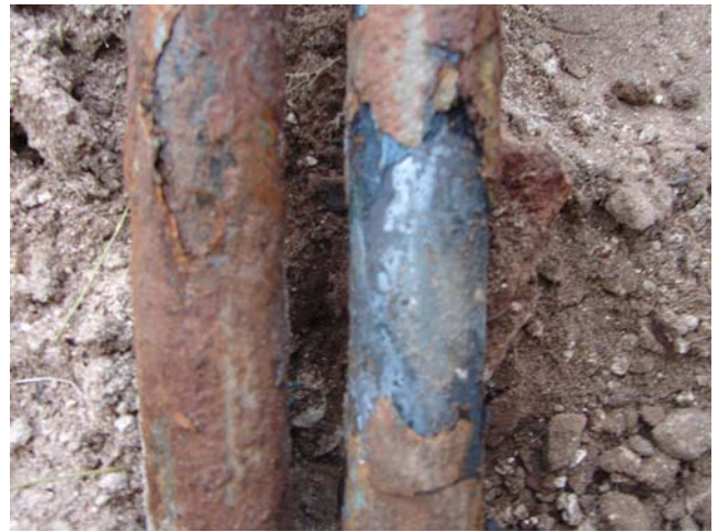
Close-up (2.5 Feet Below Ground Level)
