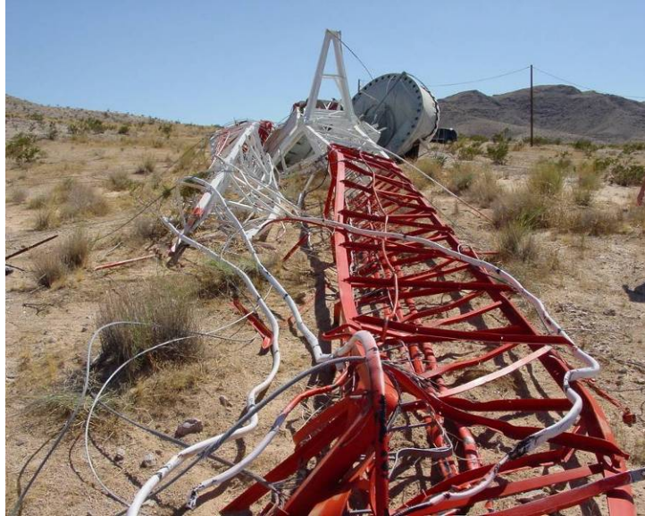
August 2005 - The collapsed tower in San Bernardino County, CA.
