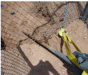
August 2005 - This tower, in Maricopa County, AZ did not collapse. Note that the condition of the anchor shaft at the surface shows no corrosion. Deterioration at two points further down the shaft show significant corrosion.
