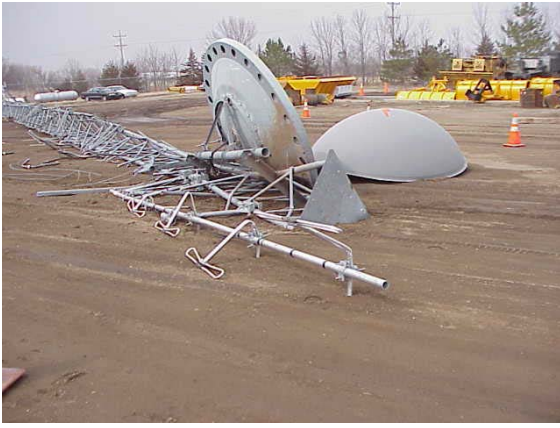
Mitchell, SD (installed 10/89, failed 3/18/2003)
