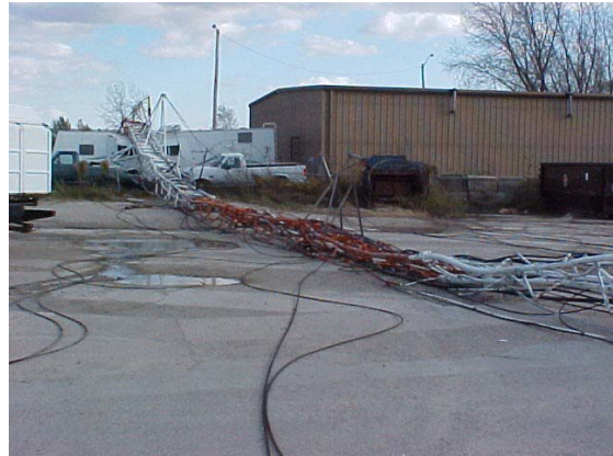
Morton, IL failed tower - 2001
